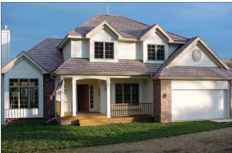
Build A Better Home research demonstration house USDA Forest Products Laboratory; Madison, Wisconsin
