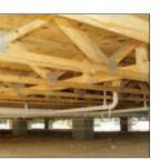
expedites construction. For example, concrete and masonry work does not have to wait on plumbing installation and inspection, which is the case with slab-on-grade construction.
