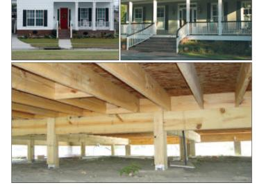
**Simple Foundation** Any foundation can settle, but a raised wood floor system makes leveling or repairs simple.
