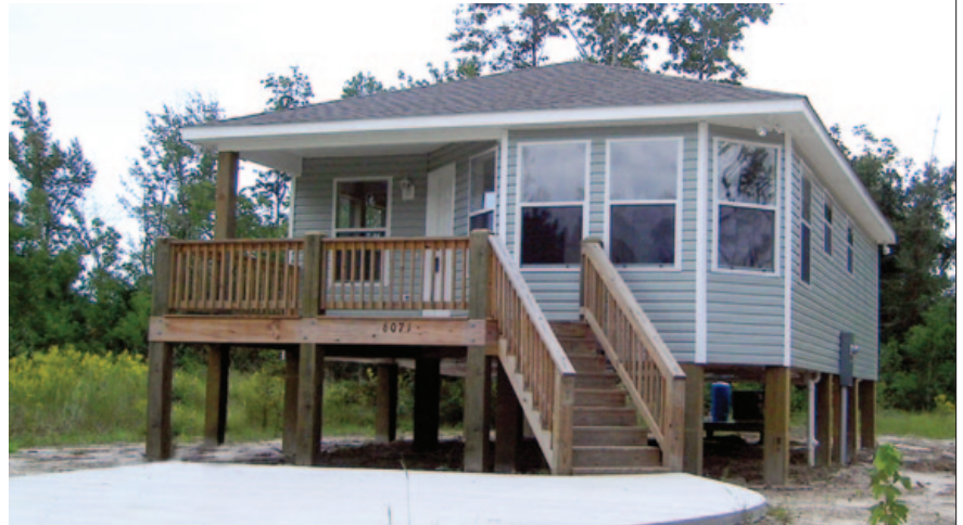
➤ Treated wood pile foundations, such as this one constructed by Bay Homes, are cost effective whether near the beach or inland.
